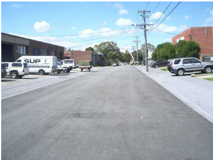
Reconstructed Industrial Roads (Beach Ave & Spray Ave)
