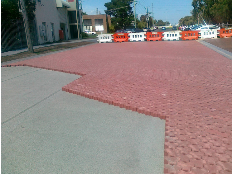
Interlock Porous Pavers (Asset Management trial on an industrial road)
