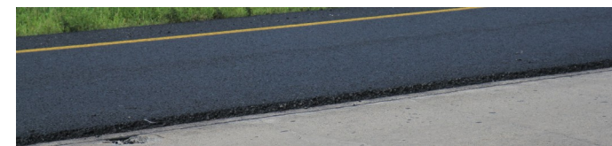
Virginia DoT - Warm Mix SMA on cracked concrete pavement
